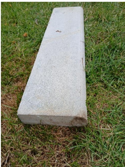
Fig 5 Edging stone. Note the rounded and square edges
